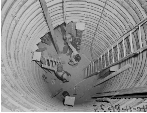
JANGLE Uncle emplacement shaft completed
